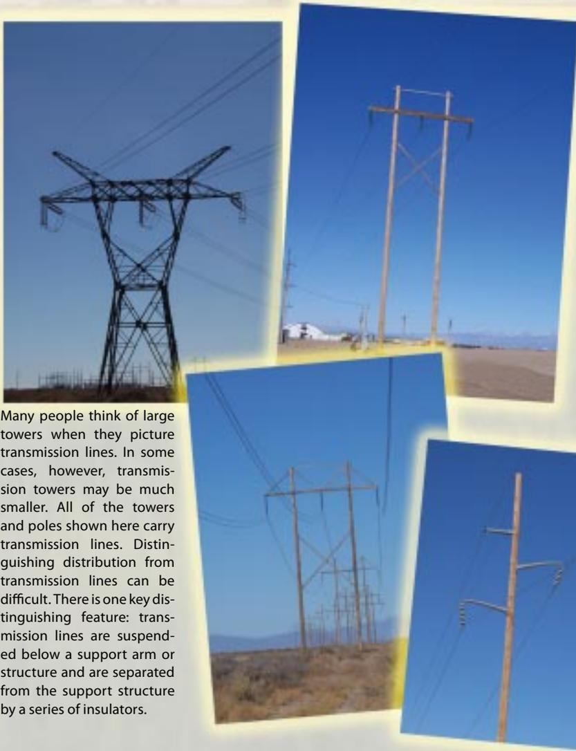
Many people think of large towers when they picture transmission lines. In some cases, however, transmission towers may be much smaller. All of the towers and poles shown here carry transmission lines. Distinguishing distribution from transmission lines can be difficult. There is one key distinguishing feature: transmission lines are suspended below a support arm or structure and are separated from the support structure by a series of insulators.
