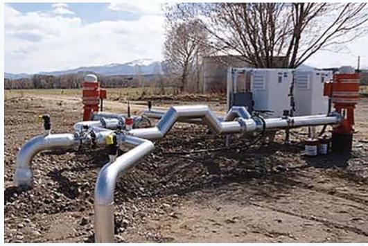
An irrigation system that maximizes use of surface water and minimizes the use of well water. The system will pay for itself in about 7 years via energy and water savings.
